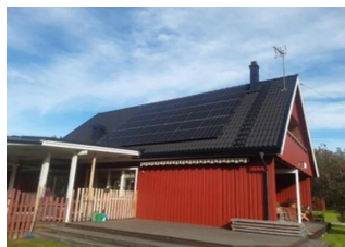
14.76KW in Sweden
