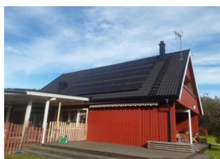
14.76KW in Sweden
